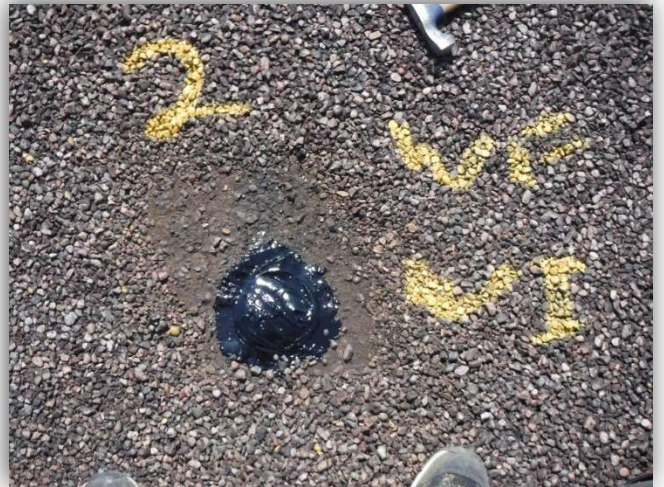
Probe #2 Roof Section 1.0
