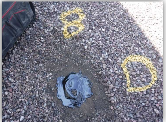
Probe #8 Roof Section 1.0
