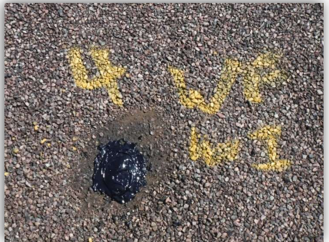
Probe #4 Roof Section 1.0
