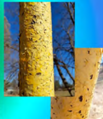
The paint on the swing posts is chipped
