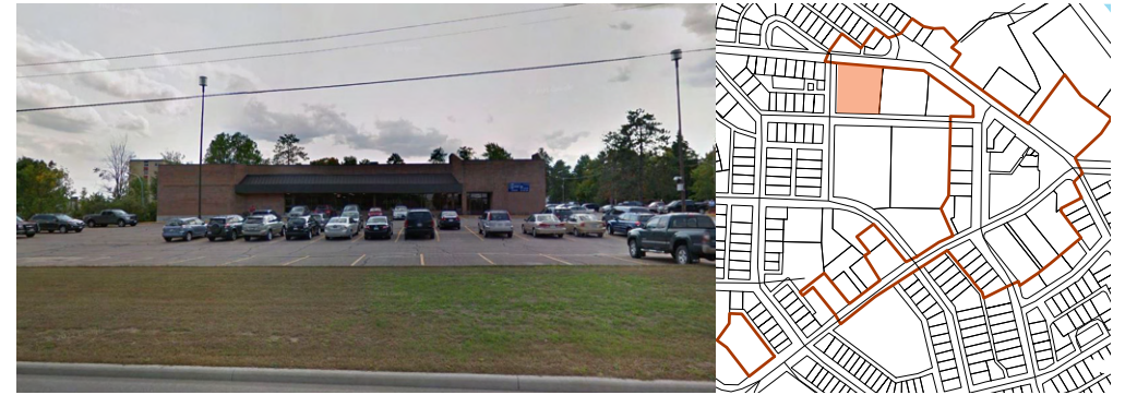
Figure 26: GC Laurence Hall on Ridge Rd.
