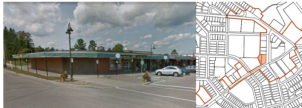
Figure 35: Commercial building and canopies on Champlain St. No openings Deep River Rd frontage.
