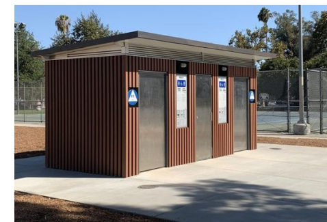
Figure 94: public washrooms reference.
