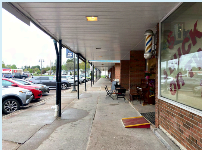
Figure 65: View of the canopies on Champlain Street. Source: Fotenn
