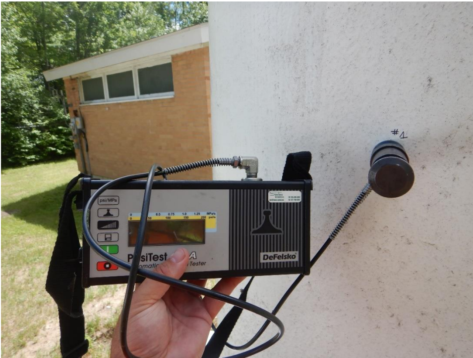
Digital Image #8. – Deep River Water Tower – DeFelsko PosiTest AT-A automatic Type V Tester used for adhesion bond strength test in ten (10) locations on the water tower legs, riser and upper bowl.
