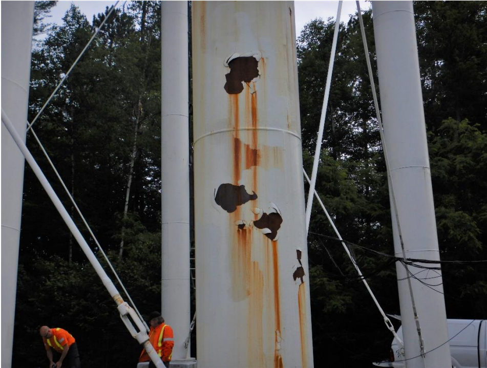
Digital Image #4. – Deep River Water Tower – The exterior coating system on the leg area of the Deep River water tower were visually inspected and at the time was found to be in poor condition with approximately 30% coatings deterioration occurring
