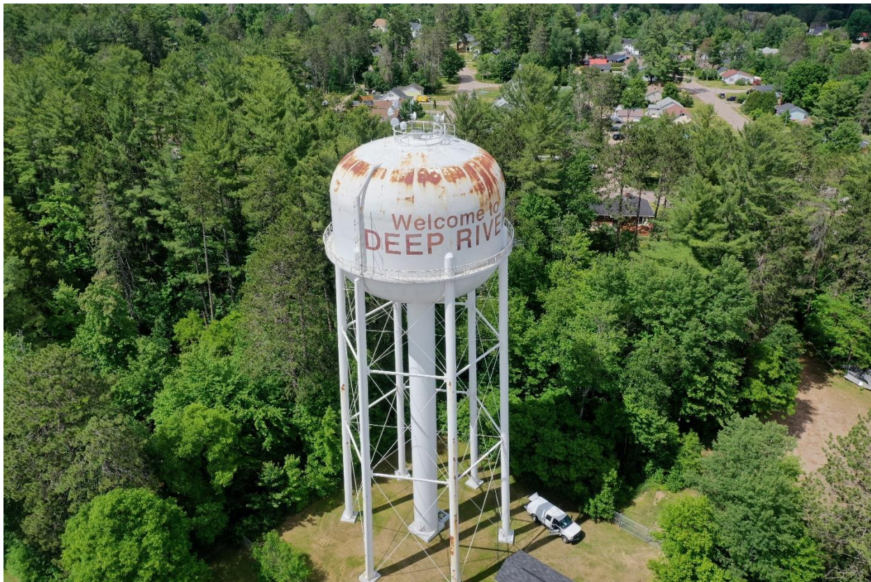
Deep River Water Tower.
