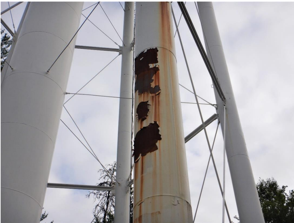
Digital Image #3. – Deep River Water Tower – The exterior coating system on the leg area of the Deep River water tower were visually inspected and at the time was found to be in poor condition with approximately 30% coatings deterioration occurring.
