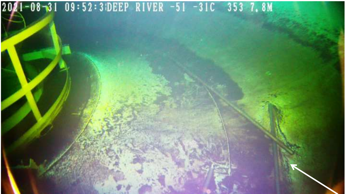
Video Image #18 – Deep River Multi-Leg Potable Water Tower – Below the Waterline – Lower Shell Area. (Video Image enhanced – brightness & Contrast, to make lining defects stand out). Center riser and floor bowl area. Bowl coating system could not be evaluated due to the sediment on the bowl floor areas. Construction material or parts of a cathodic protection system was identified on the bowl floor area.
