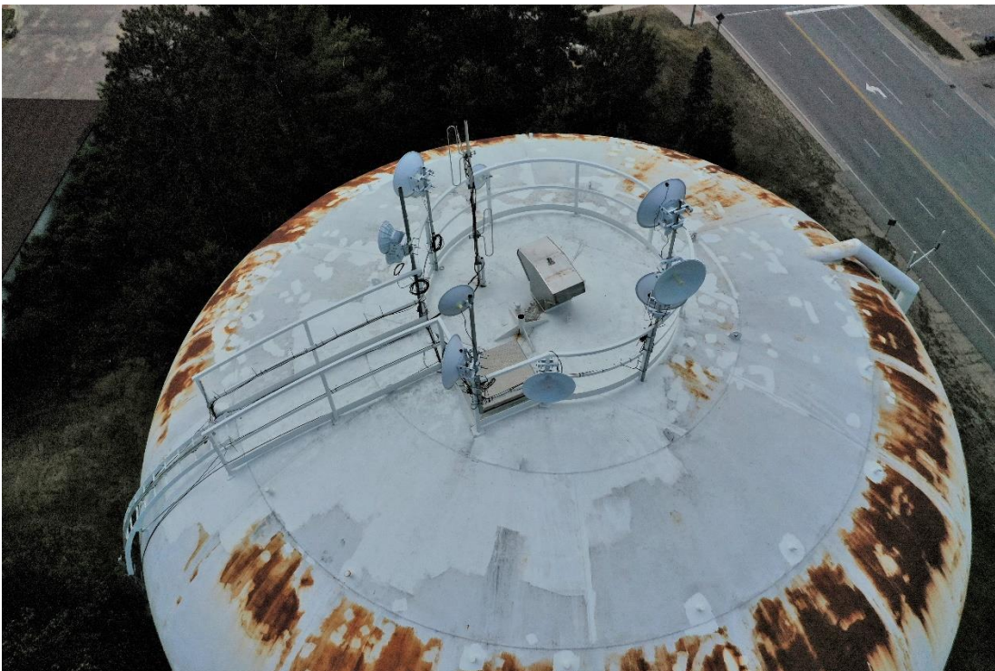
Digital Image #28. – Deep River Water Tower – Same image as above, all communication devices on the tower roof appeared to be securely attached at the time of inspection. No aircraft warning lights are on the water tower roof.
