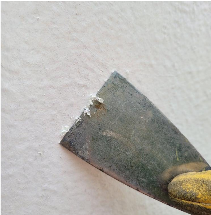
Digital Image #7. – Deep River Water Tower – There was a softening of the coating reaction to the MEK solvent, indicating the exterior coating system as being an Alkyd based coating
