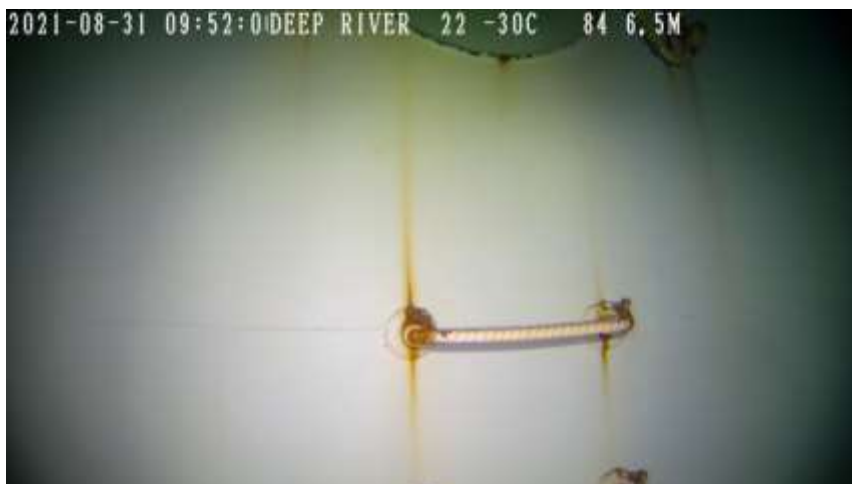
Video Image #13 – Deep River Multi-Leg Potable Water Tower – Below the Waterline – Lower Shell Area. (Video Image enhanced – brightness & Contrast, to make lining defects stand out). Generally, the lining system on the shell area of the Deep River Tower appears to be in good condition. Platform mainway ladder rungs appear to be intact at this time.
