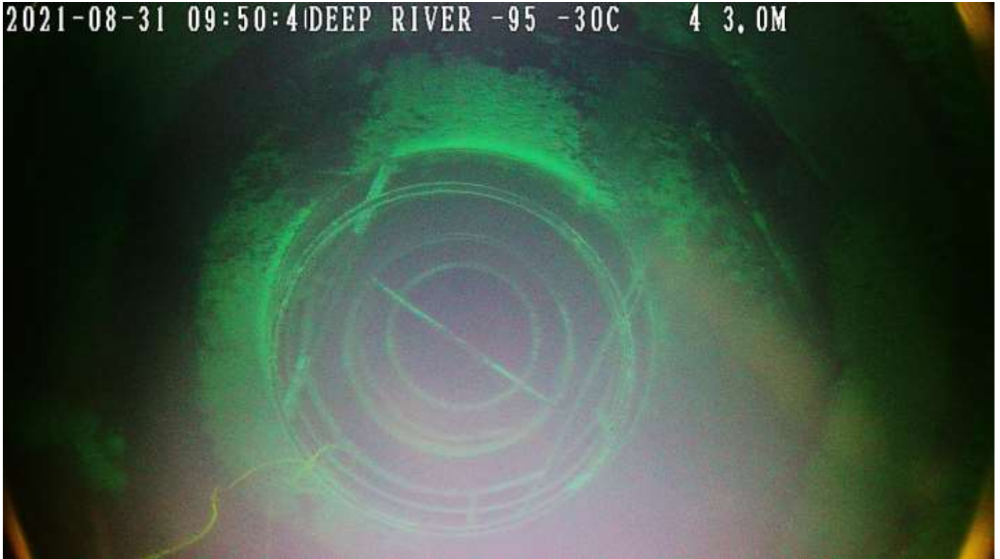
Video Image #19 – Deep River Multi-Leg Potable Water Tower – Below the Waterline – Lower Shell Area. (Video Image enhanced – brightness & Contrast, to make lining defects stand out). Center riser and floor bowl area. CCTV ROV looking down into the riser.
