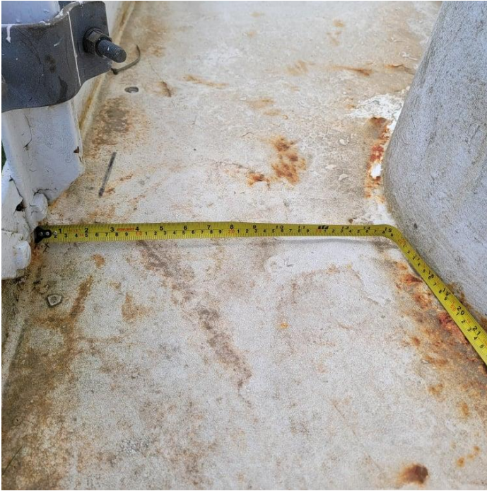
Digital Image #21. – Deep River Water Tower – The bowl platform/walkway, the access between the tower legs at the bowl and the handrailing is only 15". OH&S specifies platforms shall be at least 18" wide.
