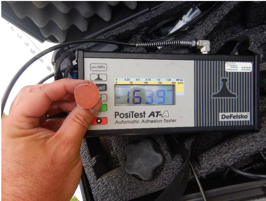
Digital Image #10. – Deep River Water Tower – Adhesion bond strength test pull results location #1 of ten (10) locations on the water tower legs, riser and upper bowl utilizing the DeFelsko PosiTect AT-A Automatic Type V Tester.
