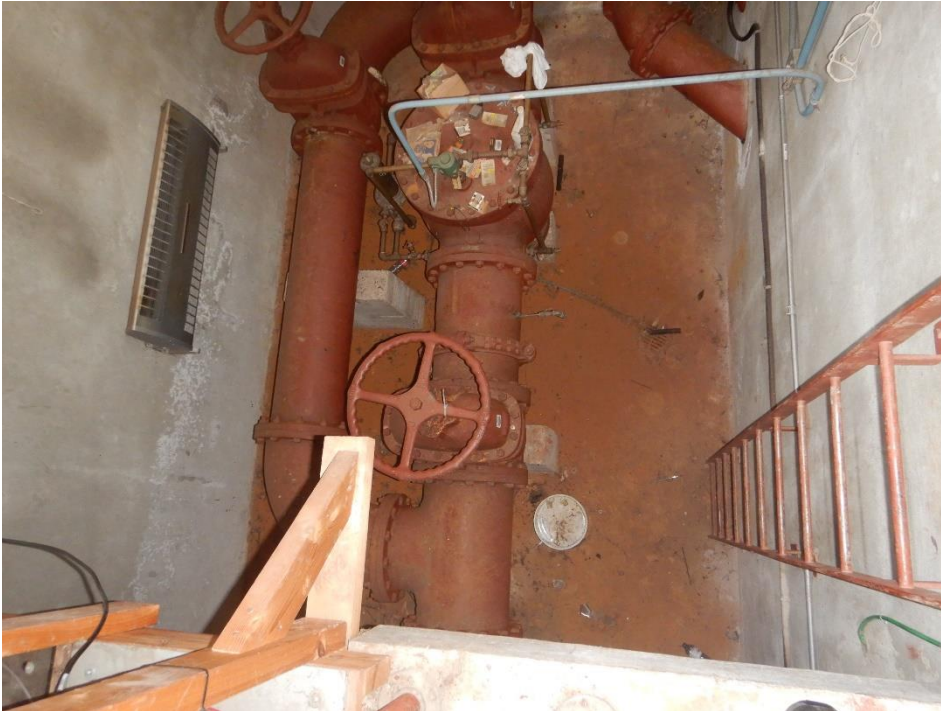
Digital Image #31. – Deep River Water Tower – The valve chamber coating system within the valve chamber has mechanical damage and corrosion occurring.
