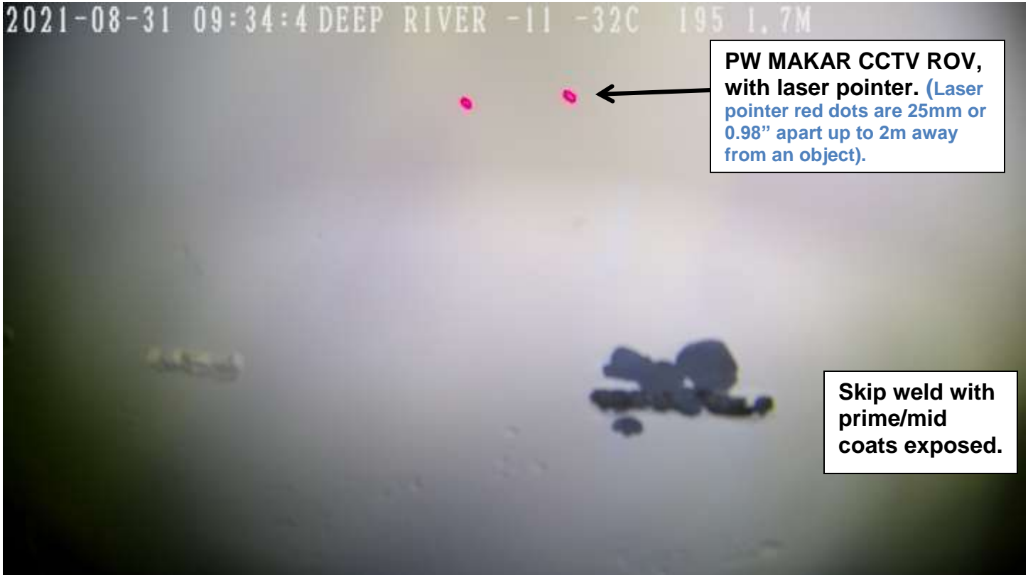
Video Image #9 – Deep River Multi-Leg Potable Water Tower – Below the Waterline – Upper Shell Area. (Video Image enhanced – brightness & Contrast, to make lining defects stand out). Generally, the lining system on the shell area of the Deep River Tower appears to be in good condition. This upper area of the shell, appears to be in the “water fluctuation zone”, where water and particularly ice builds up in the winter months and fluctuates up and down within the tower and rubs the lining system where there is protrusions. In this area, the protrusions are the weld seam and skip welds. Please note there is no rust streaking, just exposed primer and/or mid coats.
