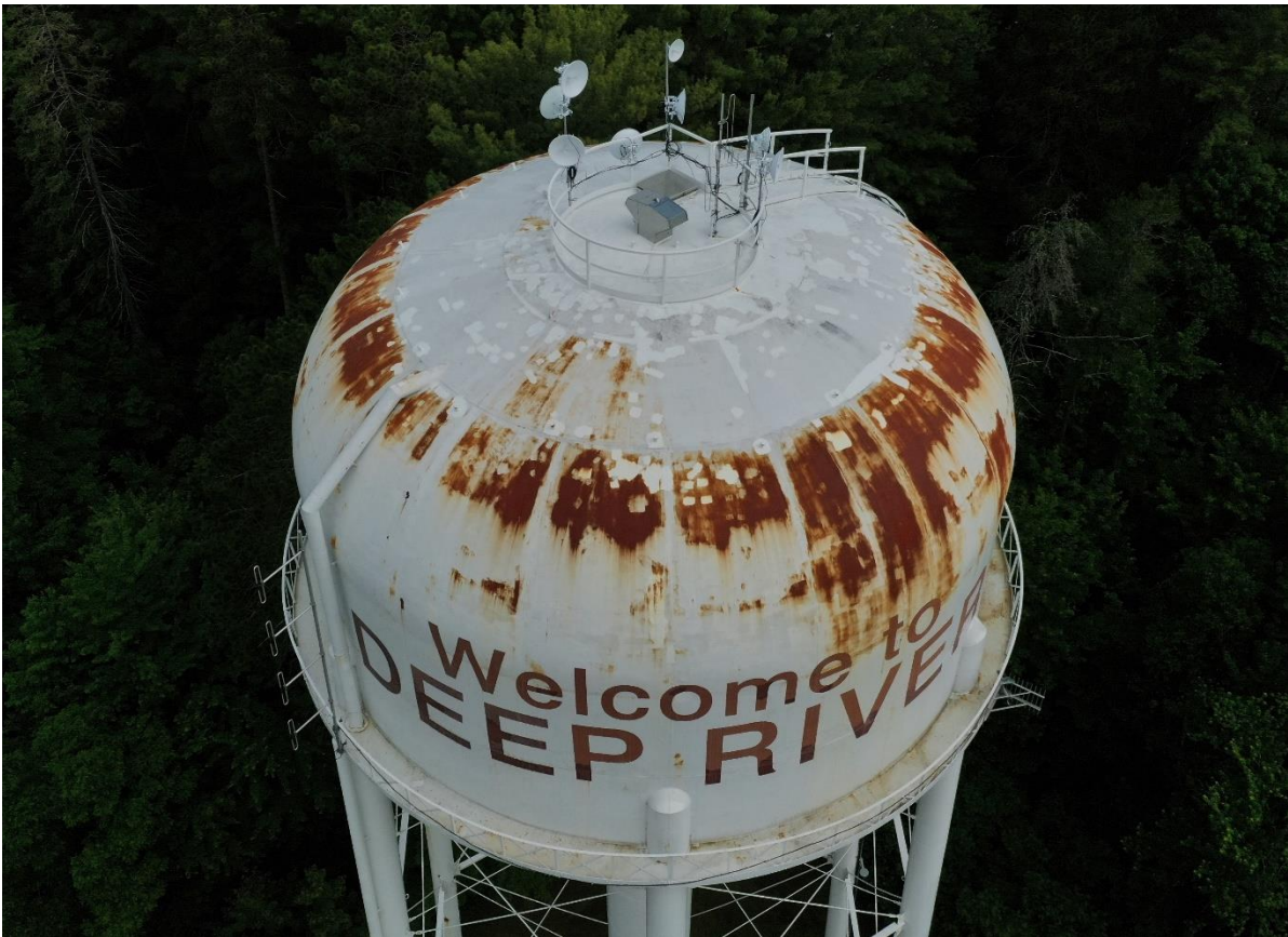
Digital Image #1. – Deep River Water Tower – The exterior coating system on the bowl area of the Deep River water tower were visually inspected and at the time was found to be in poor condition with approximately 30% coatings deterioration occurring.
