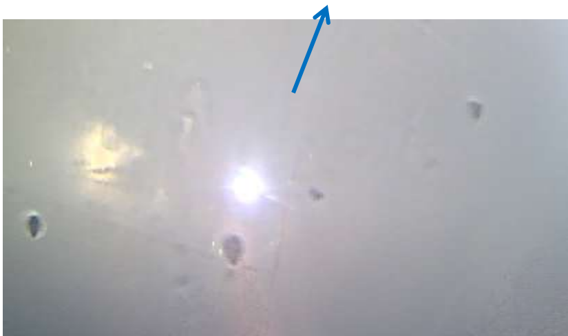
Video Image #5 – Deep River Multi-Leg Potable Water Tower – Above the water level – Roof Area. (Video Image enhanced – brightness & Contrast, to make lining defects stand out). Same as previous video image, image cropped and zoomed in. (“This writer is not assured of the dark spots on the roof area, which has been circled in blue, they may be painters swing stage nozzles or exposed primer/mid coats, since there is no rust streaking from the dark spots”).
