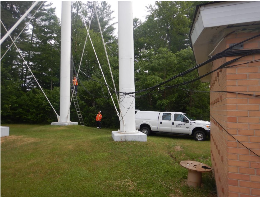
Digital Image #30. – Deep River Water Tower – Communication internet cables require cable management. Cables are tangled and hanging and are obstructing movement around the water tower grounds.
