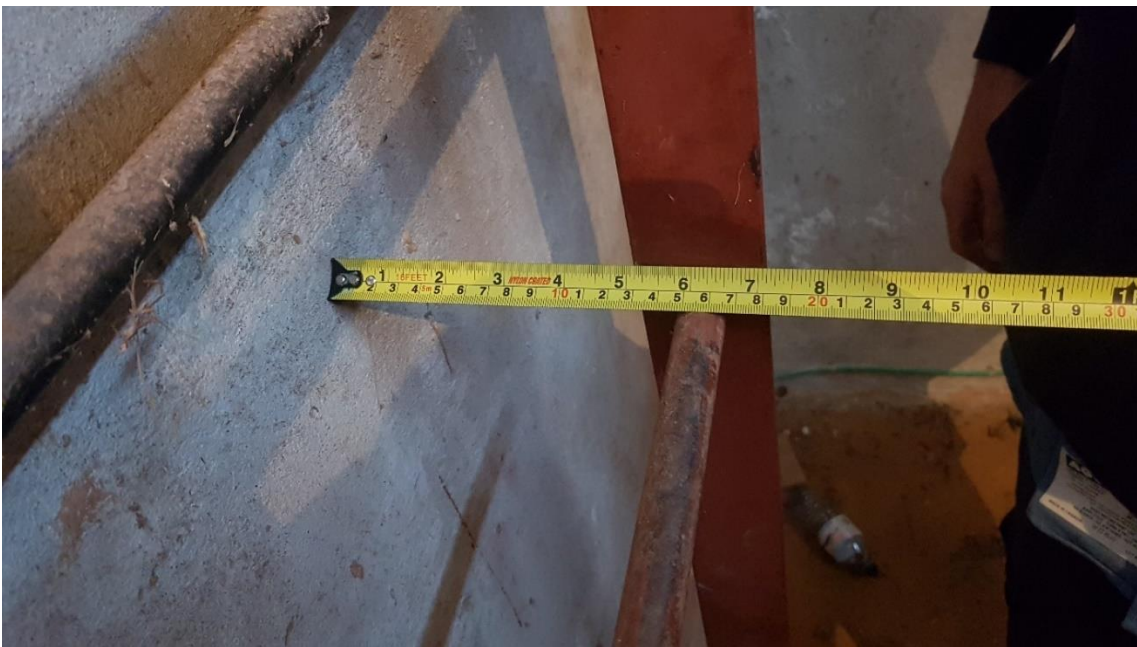
Digital Image #33. – Deep River Water Tower – The ladder rung to the chamber wall spacing on the vertical ladder is 6 1/4" total. This meets OH&S requirement of a ladder rung depth spacing total of 5.9".
