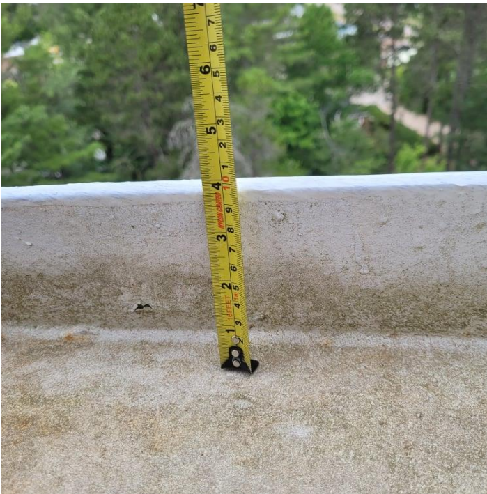
Digital Image #20. – Deep River Water Tower – The bowl platform/walkway toeboard is 4” around the entire bowl area. OH&S specifies a toeboard of 5” is required.
