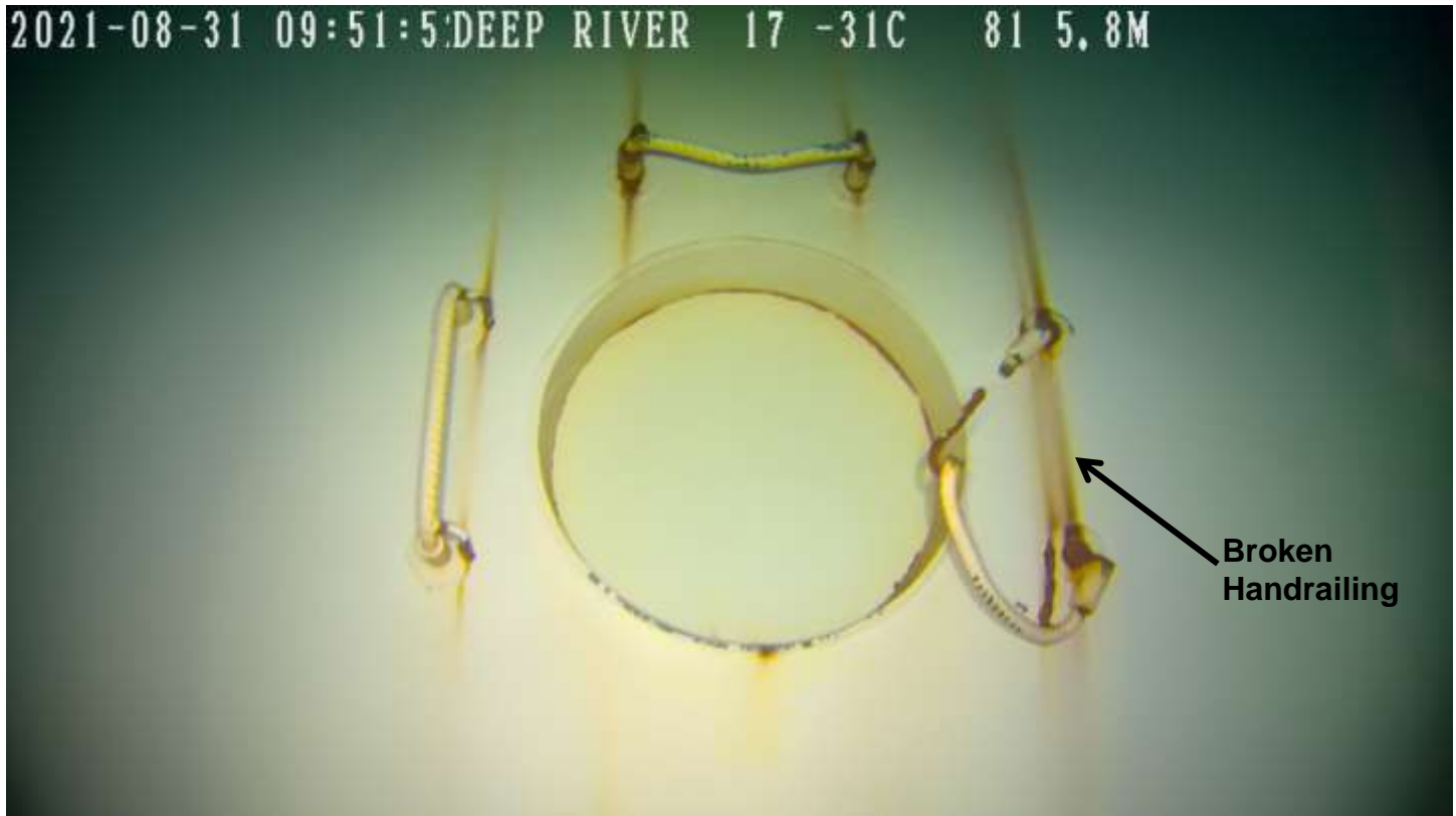
Video Image #12 – Deep River Multi-Leg Potable Water Tower – Below the Waterline – Lower Shell Area. (Video Image enhanced – brightness & Contrast, to make lining defects stand out). Generally, the lining system on the shell area of the Deep River Tower appears to be in good condition. Rust streaking from platform manway access handrailings. Note, on the right side of the manway, the handrailing is broken.
