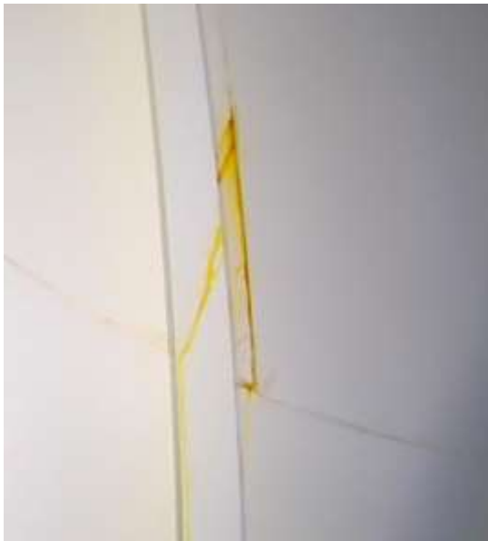
Video Image #3 – Deep River Multi-Leg Potable Water Tower – Above the Waterline – Roof Area. (Video Image enhanced – brightness & Contrast, to make lining defects stand out). Same as previous video image, image cropped and zoomed in. Rust present on roof weld seam.
