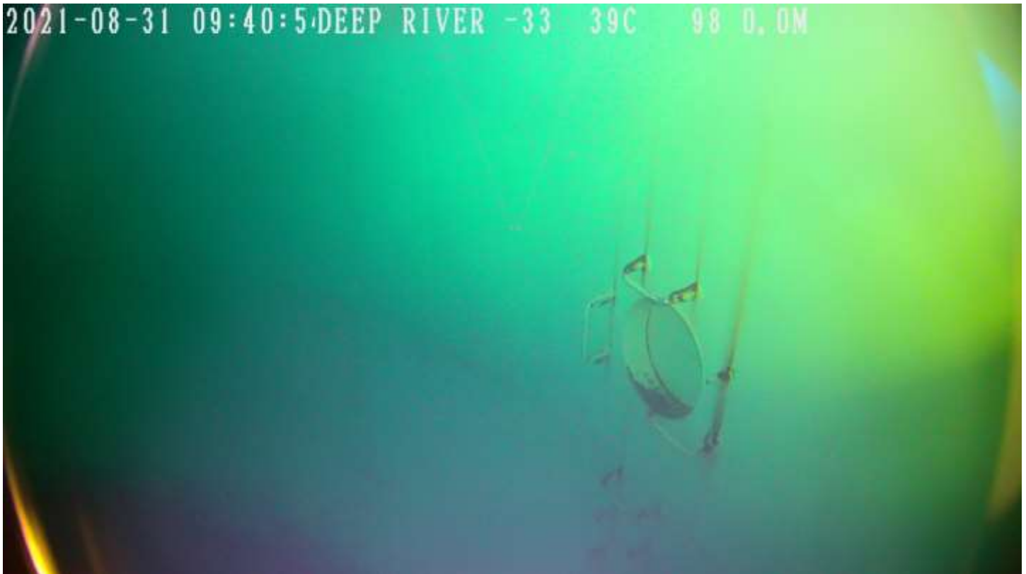
Video Image #11 – Deep River Multi-Leg Potable Water Tower – Below the Waterline – Lower Shell Area. (Video Image enhanced – brightness & Contrast, to make lining defects stand out). Generally, the lining system on the shell area of the Deep River Tower appears to be in good condition. Rust streaking from Platform Manway access handrailings. Note, on the right side of the manway, the handrailing is broken.
