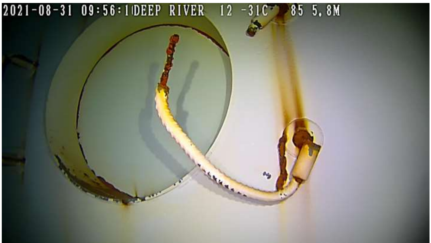
Deep River – Multi-Leg Potable Water Tower – Shell Area – Broken Platform Manway Access Handrailing.
