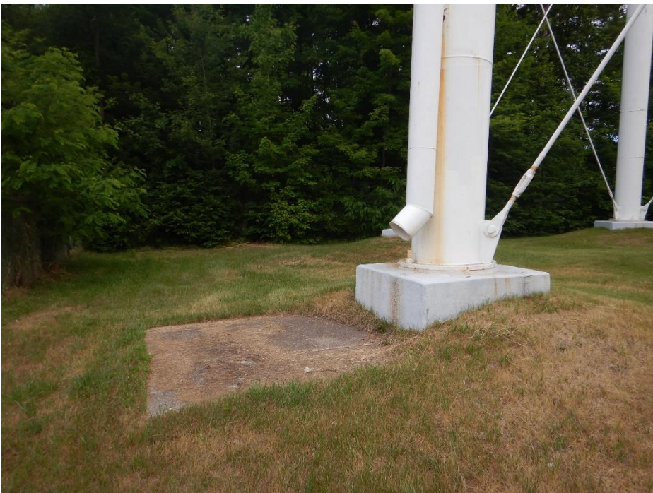
Digital Image #12. – Deep River Water Tower – The tower leg concrete base pad and drainpipe pad are in good condition with only small amounts of visible weathering and small cracking visible. Drainpipe is recommended to be extended to avoid future deterioration of leg concrete base pad.
