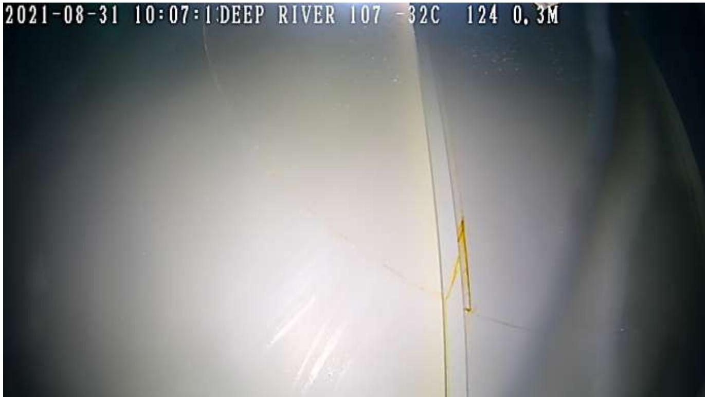
Video Image #2 – Deep River Multi-Leg Potable Water Tower – Above the Waterline – Roof Area. (Video Image enhanced – brightness & Contrast, to make lining defects stand out). The lining system on the roof area of the Deep River Tower appears to be in good condition, with a few very minor isolated areas of spot rust streaking apparent at this time.
