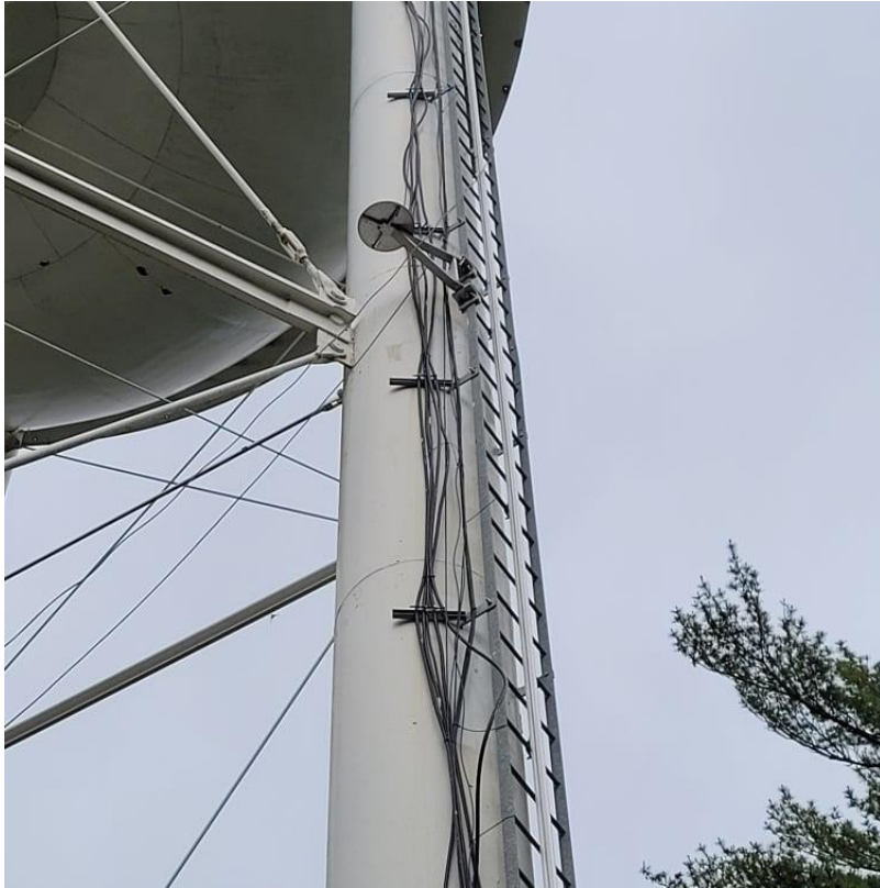
Digital Image #17. – Deep River Water Tower – Internet communication cables are attached to the ground to bowl ladder and obstruct the ladder and the safety rest seats and is recommended to be affixed in a clean manner that will not obstruct access and egress.
