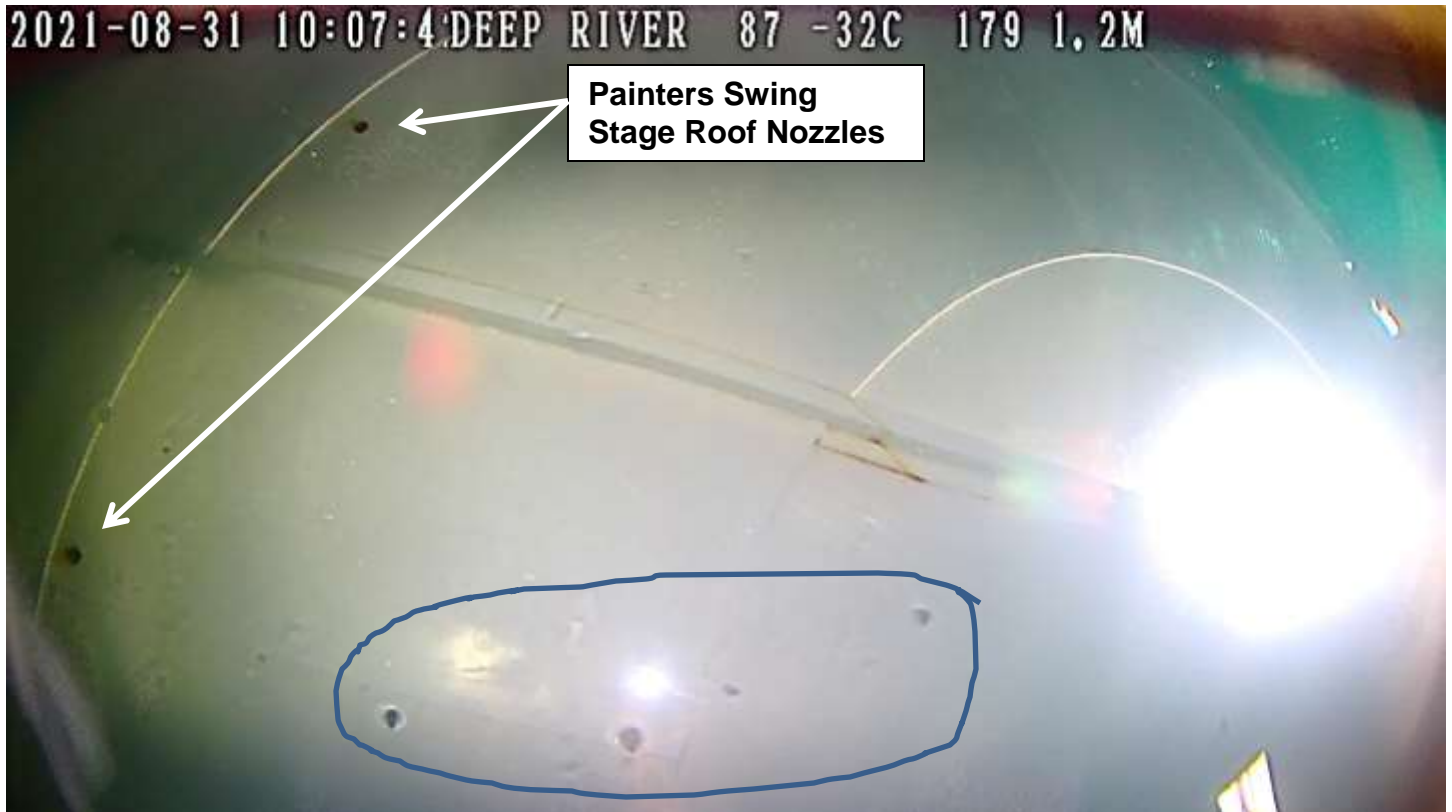
Video Image #4 – Deep River Multi-Leg Potable Water Tower – Above the water level – Roof Area. (Video Image enhanced – brightness & Contrast, to make lining defects stand out). A few very minor isolated areas of spot rust streaking appeared at this time. (“This writer is not assured of the dark spots on the roof area, which has been circled in blue, they may be painters swing stage nozzles or exposed primer/mid coats since there is no rust streaking from the dark spots”).
