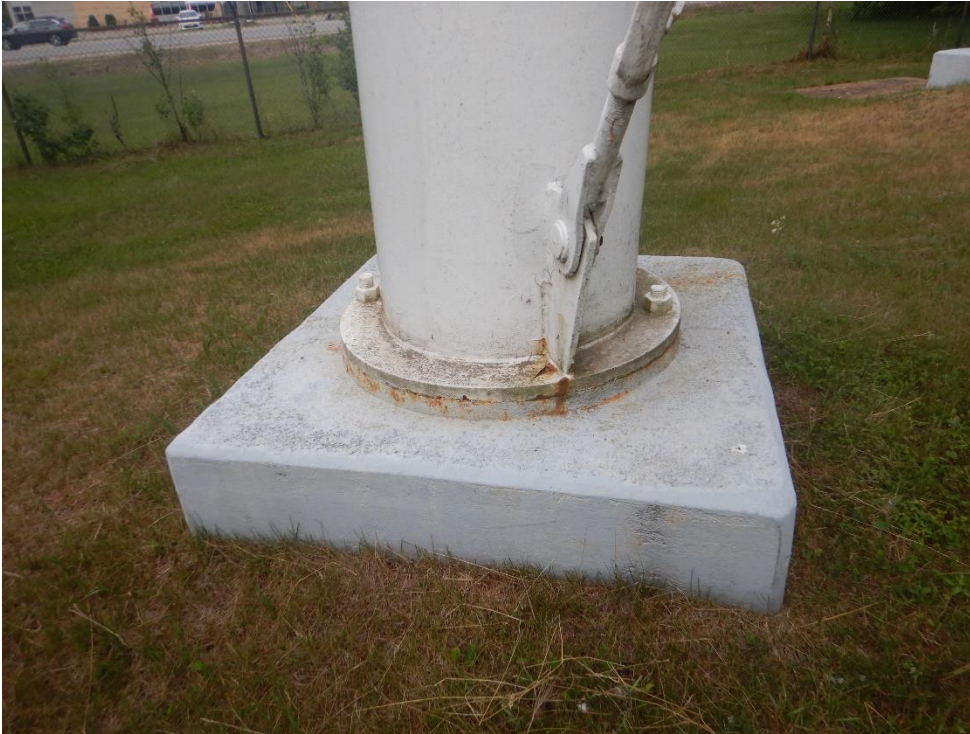
Digital Image #11. – Deep River Water Tower – The tower leg concrete base pads and riser base pad are in good condition with only small amounts of visible weathering and small cracking visible.
