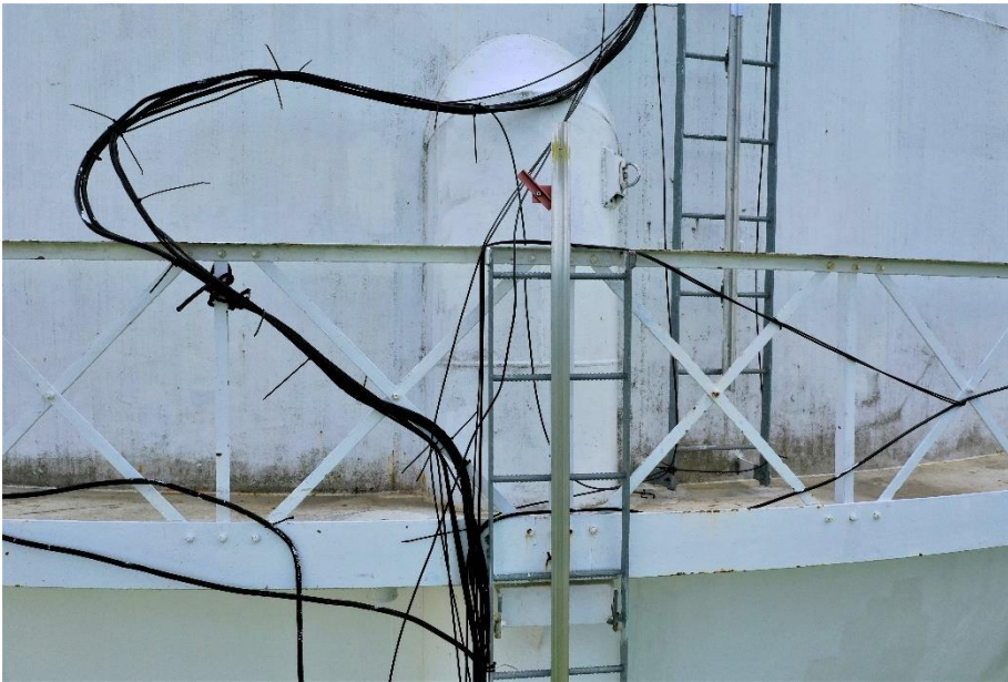
Digital Image #18. – Deep River Water Tower – Internet communication cables hindered the access and egress to the bowl walkway/platform as well as the placement of the walkway handrail, toeboard, extended aluminum ridge rail and fall arrest system.
