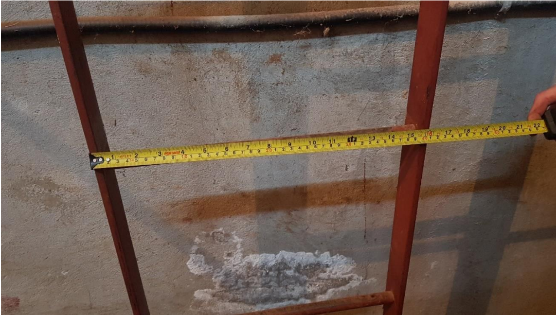
Digital Image #32. – Deep River Water Tower – The valve chamber ladder width of the ladder rungs is 16". OH&S specifies a ladder rung spacing total of 23.6".
