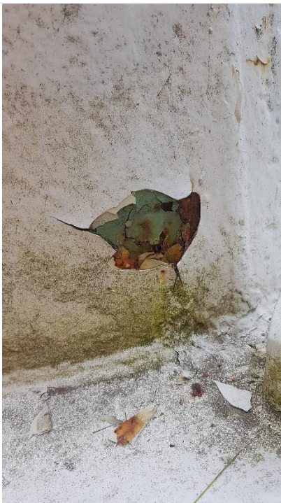
Digital Image #5. – Deep River Water Tower – The exterior coating system on the Deep River water tower appeared to have 6 layers of previous coatings applied.
