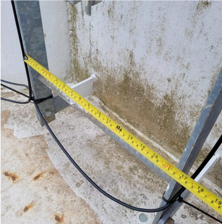
Digital Image #15. – Deep River Water Tower – The ladder from the platform/walkway to the bowl roof width of the ladder rungs is 16”, which includes the 2 ¼ “aluminum ridge rail, fall arrest system. OH&S specifies a ladder rung spacing total of 23.6”.
