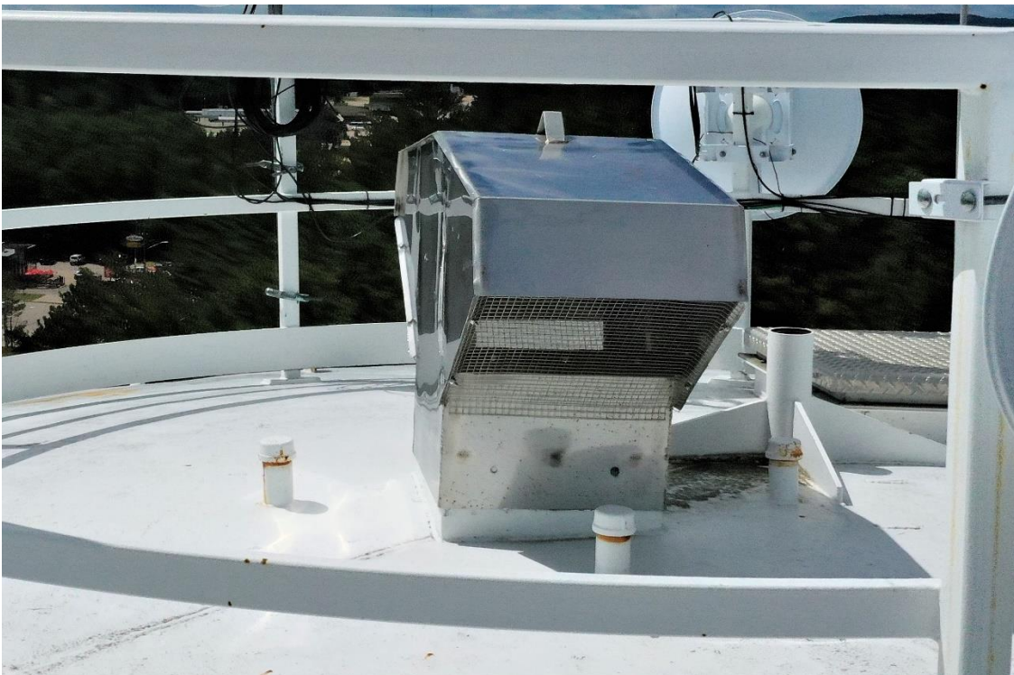
Digital Image #26. – Deep River Water Tower – The bowl roof air vent is in good condition at the time of inspection.
