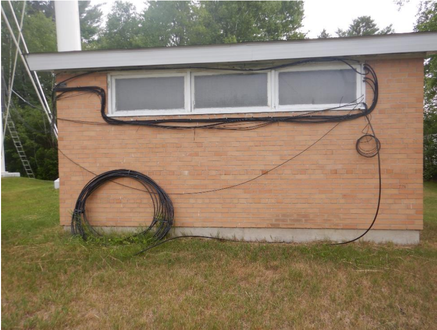
Digital Image #29. – Deep River Water Tower – Communication / Valve chamber house in good condition at the time of inspection. Internet cable management is required.
