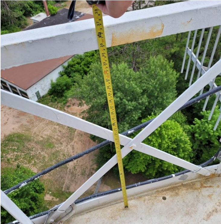
Digital Image #19. – Deep River Water Tower – The bowl platform/walkway handrail height around the tower bowl is 37” in total height. OH&S specifies a hand railing height of 35”.
