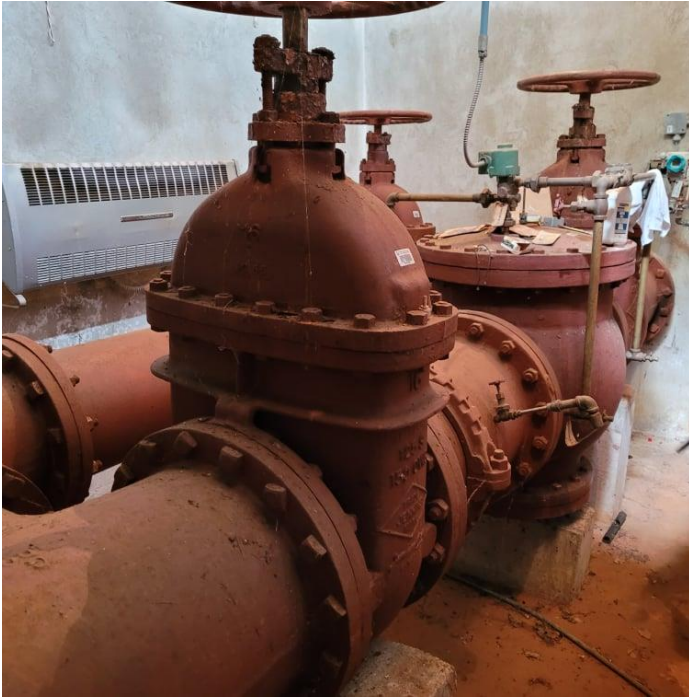
Digital Image #34. – Deep River Water Tower – The valve chamber coating system within the valve chamber has mechanical damage and deep corrosion occurring.
