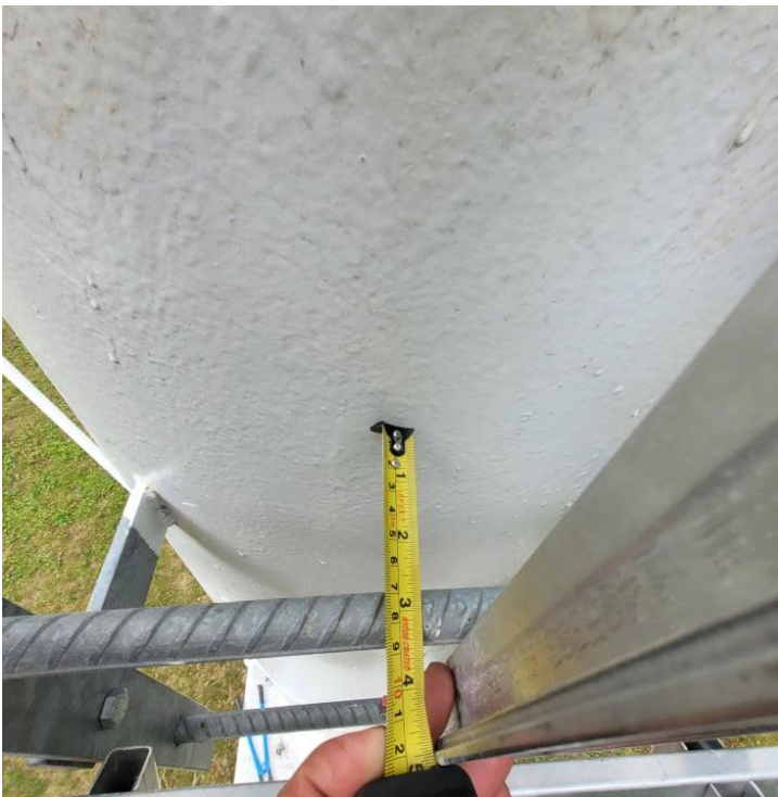
Digital Image #16. – Deep River Water Tower – The ladder rung to the water tower leg spacing on the vertical ladder from the ground to the platform/walkway is 3” total. OH&S specifies a ladder rung depth spacing total of 5.9”.
