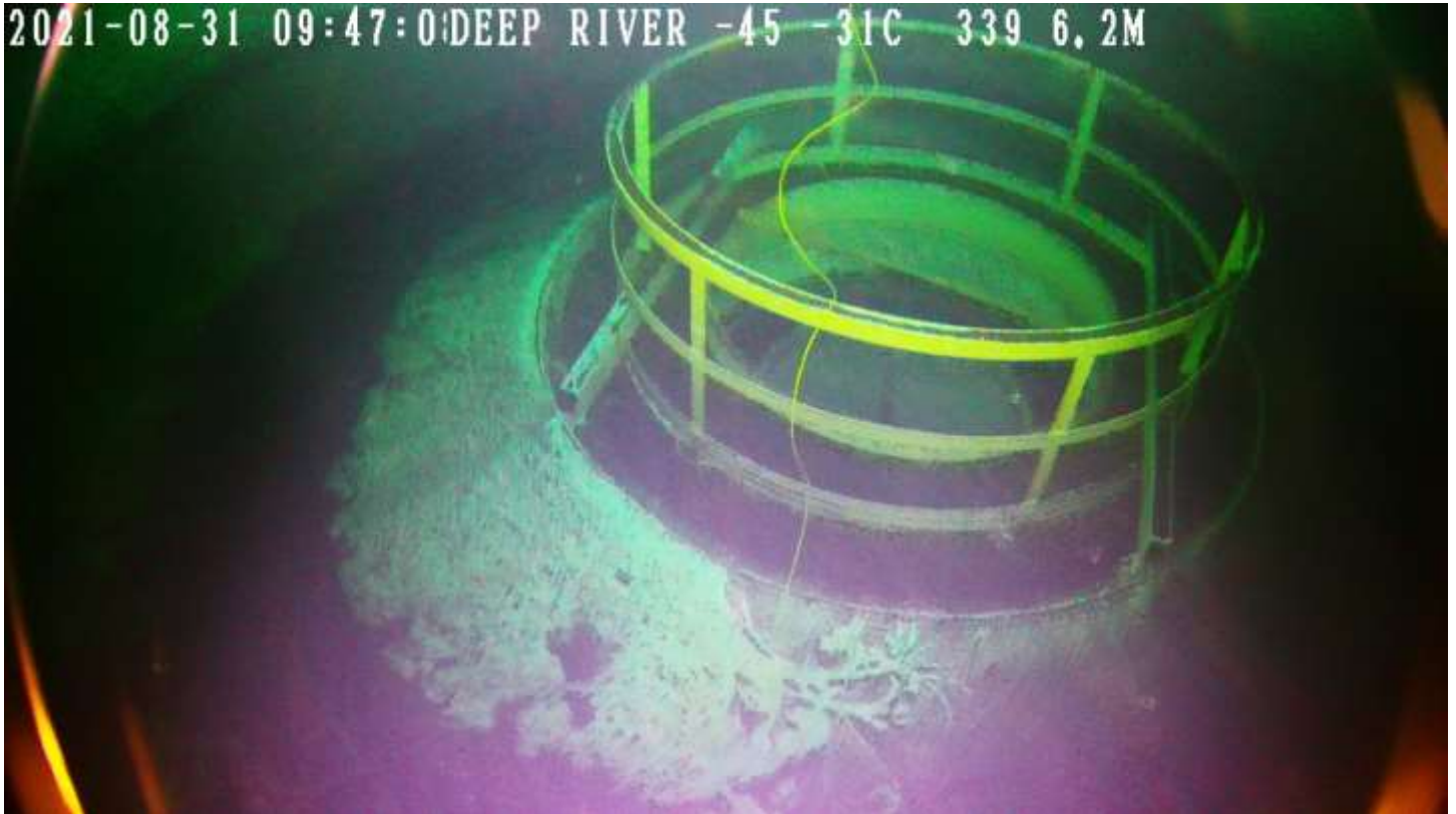
Video Image #16 – Deep River Multi-Leg Potable Water Tower – Below the Waterline – Lower Shell Area. (Video Image enhanced – brightness & Contrast, to make lining defects stand out). Center riser and floor bowl area. Bowl coating system could not be evaluated due to the sediment on the bowl floor areas. Construction material or parts of a cathodic protection system was identified on the bowl floor area.
