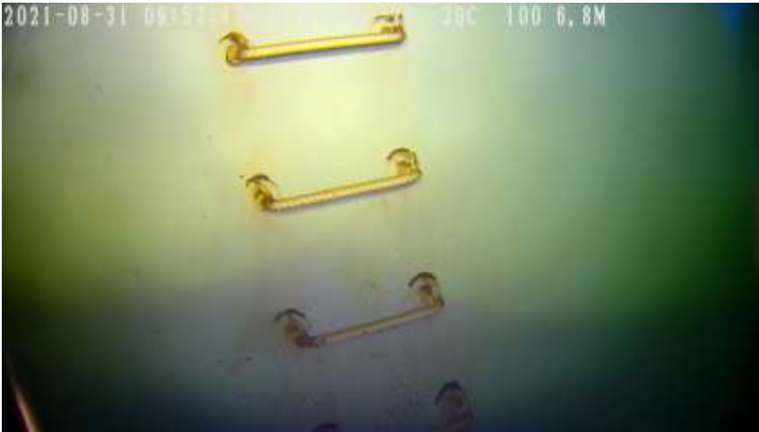
Video Image #14 – Deep River Multi-Leg Potable Water Tower – Below the Waterline – Lower Shell Area. (Video Image enhanced – brightness & Contrast, to make lining defects stand out). Generally, the lining system on the shell area of the Deep River Tower appears to be in good condition. Same as previous video image. Platform mainway ladder rungs appear to be intact at this time.
