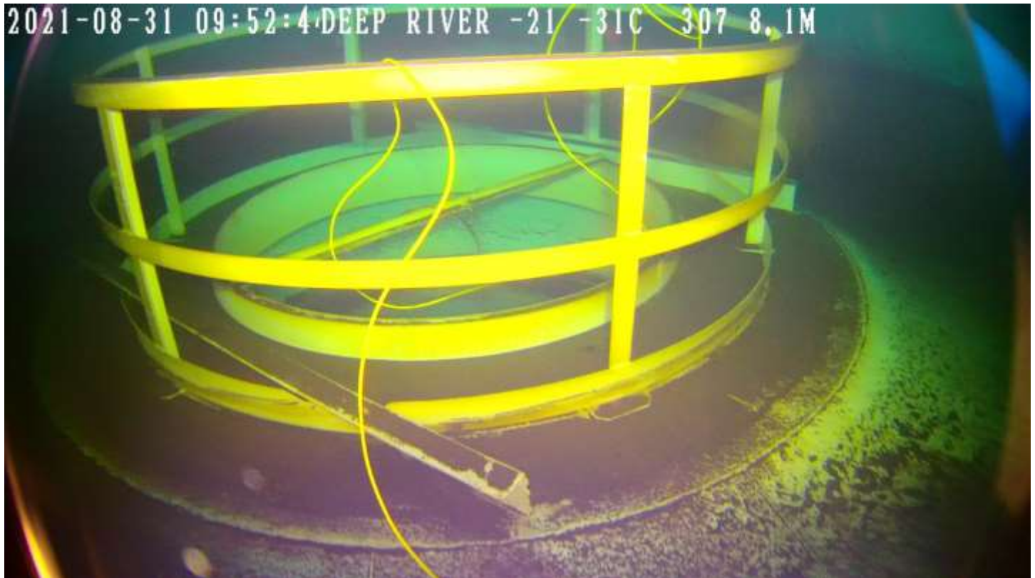
Video Image #17 – Deep River Multi-Leg Potable Water Tower – Below the Waterline – Lower Shell Area. (Video Image enhanced – brightness & Contrast, to make lining defects stand out). Center riser and floor bowl area. Bowl coating system could not be evaluated due to the sediment on the bowl floor areas. Construction material or parts of a cathodic protection system was identified on the bowl floor area.
