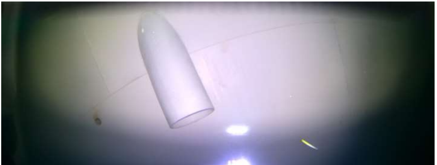
Video Image #7 – Deep River Multi-Leg Potable Water Tower – Above the Waterline – Roof Area. (Video Image enhanced – brightness & Contrast, to make lining defects stand out). Same as previous video image, image cropped and zoomed in.
