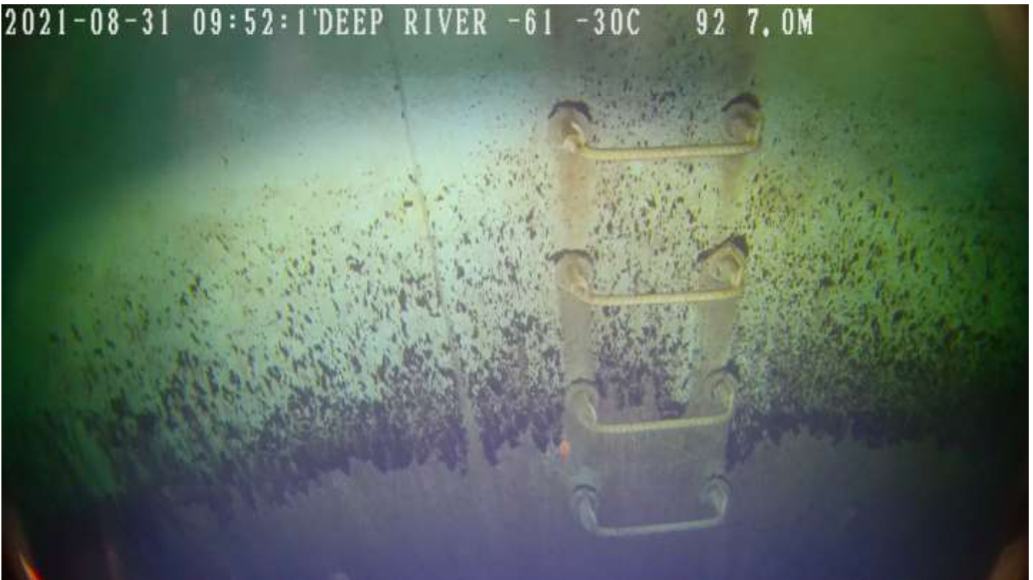
Video Image #15 – Deep River Multi-Leg Potable Water Tower – Below the Waterline – Lower Shell Area. (Video Image enhanced – brightness & Contrast, to make lining defects stand out). Generally, the lining system on the shell area of the Deep River Tower appears to be in good condition. Same as previous video image. Platform mainway ladder rungs appear to be intact at this time. Note the sediment from the bowl area.
