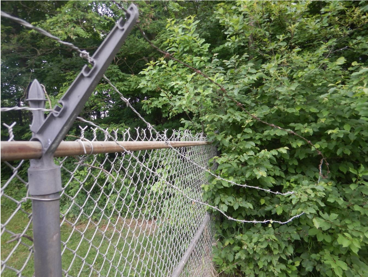
Digital Image #36. – The fence line was inspected and the 3-level barb wire security wire needs to be repaired to maximize security around the water tower.
