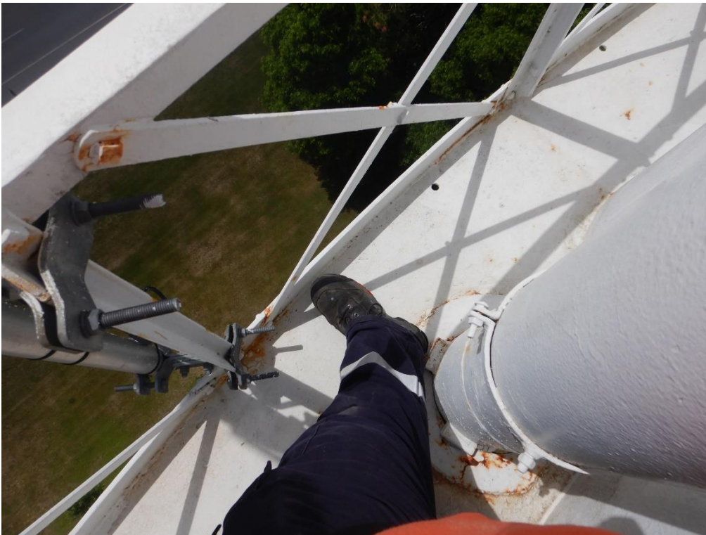
Digital Image #22. – Deep River Water Tower – The bowl platform/walkway, the access between the drainpipe and the handrailing is only 12". OH&S specifies platforms shall be at least 18" wide.
