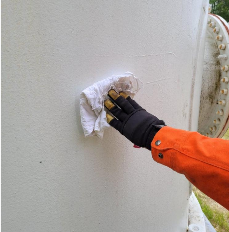
Digital Image #6. – Deep River Water Tower – A cloth rag saturated with MEK solvent was held to the surface of the water tower roof. The rag was removed and the white topcoat was tested for its hardness.
