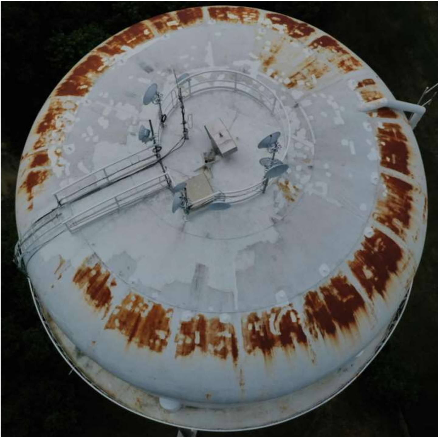
Aerial Drone Image #2 – Deep River Multi-Leg Potable Water Tower – Exterior – Roof Area. (Video Image enhanced – brightness & Contrast, to make lining defects stand out). Same as previous image. Discription of exterior roof accessories.
