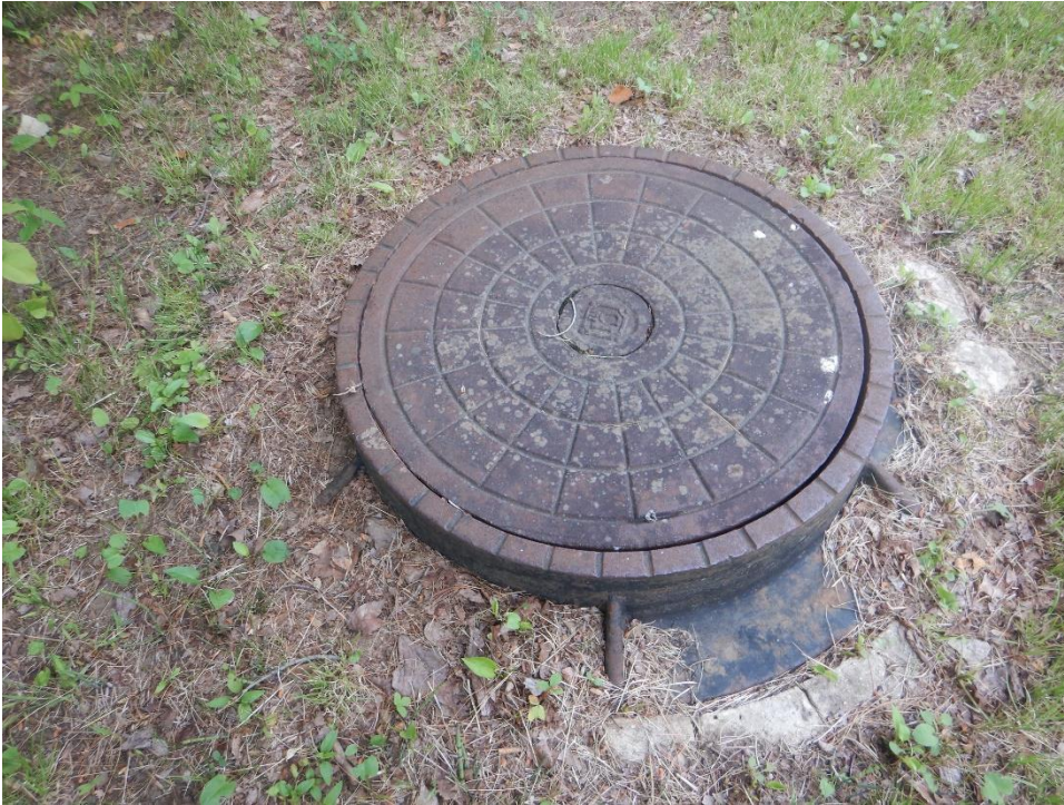
Digital Image #13. – Deep River Water Tower – Two stormwater manways are on the grounds of the tower and are in good condition.
