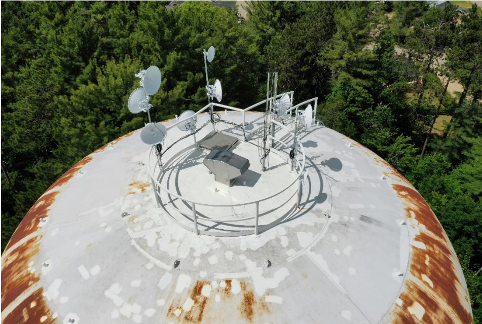
Digital Image #2. – Deep River Water Tower – The exterior coating system on the bowl area of the Deep River water tower were visually inspected and at the time was found to be in poor condition with approximately 30% coatings deterioration occurring.
