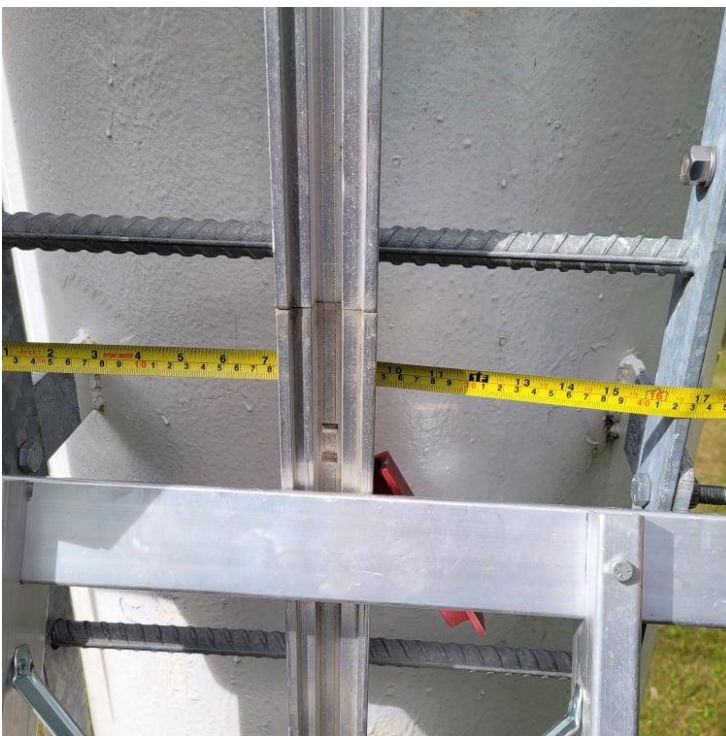
Digital Image #14. – Deep River Water Tower – The ladder to the bowl width of the ladder rungs is 16", which includes the 2 ¼ "aluminum ridge rail, fall arrest system. OH&S specifies a ladder rung spacing total of 23.6".
