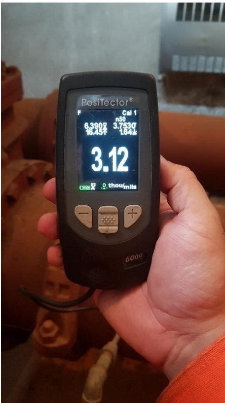
Digital Image #35. – Deep River Water Tower – Fifty (50) dry film thickness readings were taken on the pipeline of the Deep River Water Tower in the valve chamber with PosiTector 6000. The average DFT was 6.39 mils.
