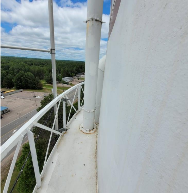
Digital Image #23. – Deep River Water Tower – Same image as above, the bowl platform/walkway, the access between the drainpipe and the handrailing is only 12". OH&S specifies platforms shall be at least 18" wide.
