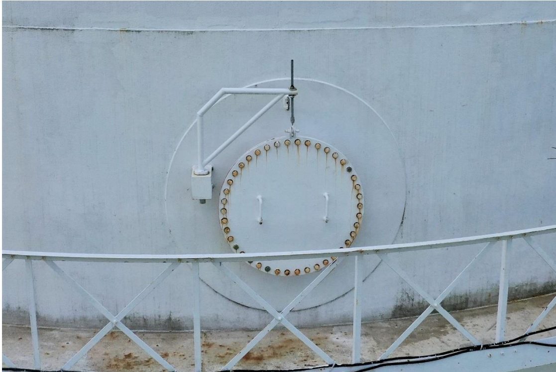
Digital Image #25. – Deep River Water Tower – The platform/walkway manway is 26” in diameter. OH&S requires a 30” manway.
