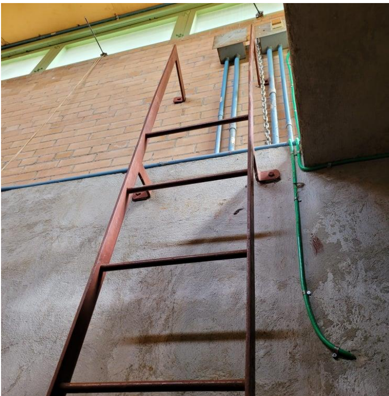
Digital Image #32. – Deep River Water Tower – The valve chamber ladder has no D-Ring at the top of the ladder or fall arrest system in place.
