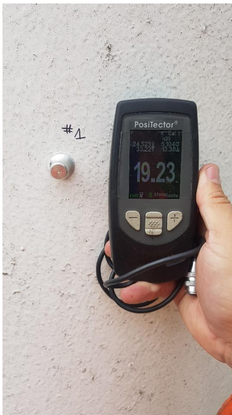
Digital Image #10. – Deep River Water Tower – Two hundred (200) dry film thickness readings were taken on the exterior of the Deep River Water Tower with PosiTector 6000. The average DFT was 23.60 mils.
