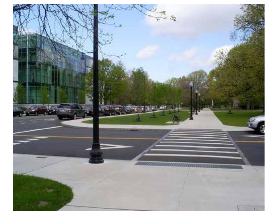
Reference Image. Source: National Association of City Transportation Officials.
