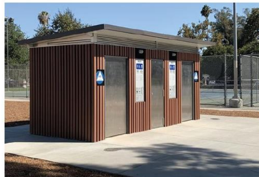
Figure 94: public washrooms reference.
