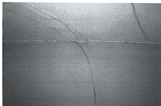
Roof to Wall Overlapping Steel Plating
