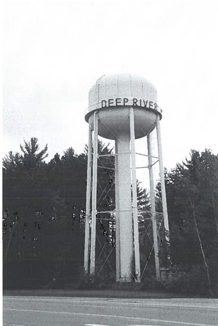
330,000 Gallon Capacity, Six Legged Structure, Elevated Tank
